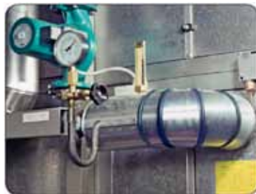
Repair on dirty surfaces
