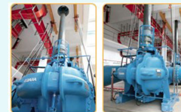
Vertical Axial Split Casing pump Suitable for Sea Water ( Full SS316 / Duplex SS ) Available with Universal Joint Shaft
