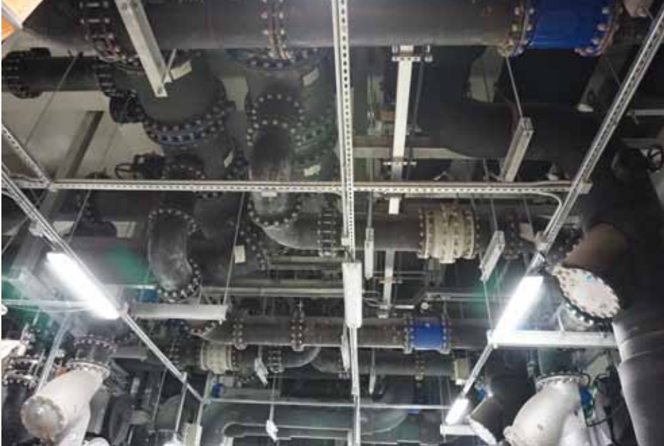
Pipe module in Chiller Building
