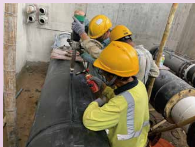
Figure 5. Electro-fusion Joint for PU Foaming
