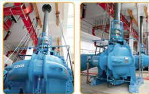
Vertical Axial Split Casing pump Suitable for Sea Water ( Full SS316 / Duplex SS ) Available with Universal Joint Shaft
