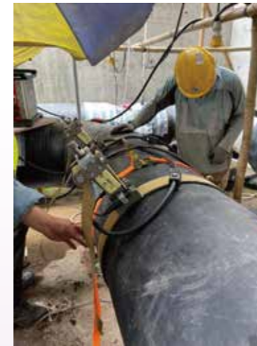
Figure 6. Electro-fusion Joint for HDPE Welding
