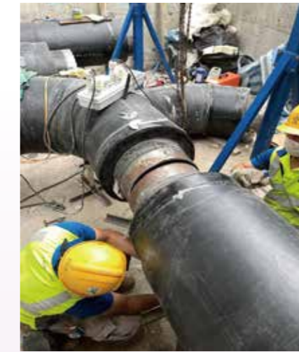
Figure 7. U/G Pipe Welding
