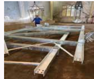
Metal Frame was prefabricated at off-site warehouse
