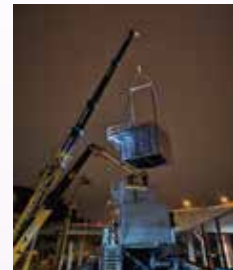
2-pieces DfMA Marley Cooling Tower at Ho Tung Lau Depot
