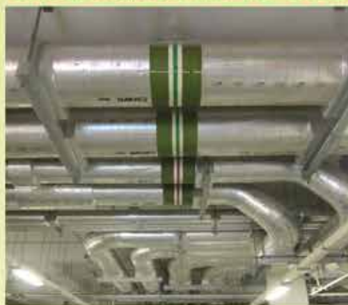
Sheet Metal Ductwork Insulation
