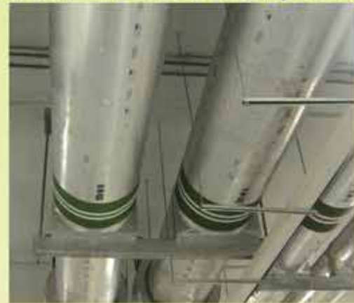
Chilled Water Pipework Insulation
