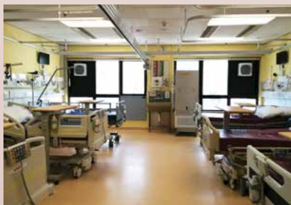
▲ Fast track conversion of Tier 2 isolation room from hospital general ward with HEPA exhaust units
