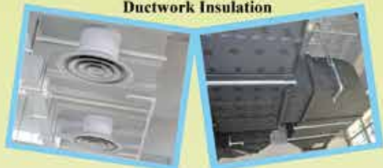
Duct Support Insulation (DSI)
